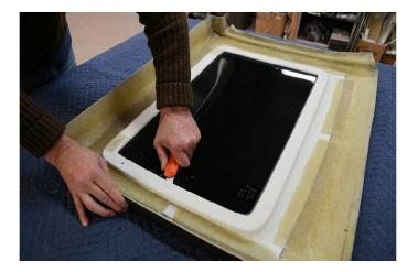
Since some force will be required to cut the tough adhesive, be very careful with the sharp knife. A slip of the knife could be very dangerous if your free hand is in the path of the slipping knife.
