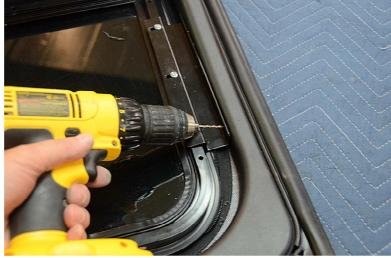
Step 7: Drive screws into the holes drilled in the previous step. Because of the position of the screws, a 1/4" open end or box end wrench may be easier to use for this step than the nut driver.
